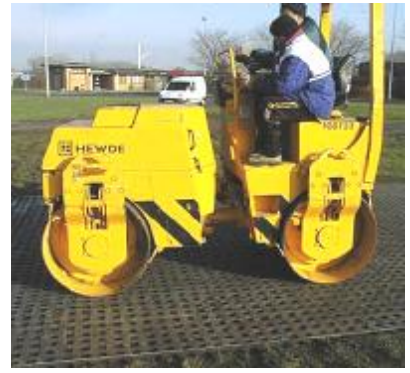
After about 3-4 rows are laid out, they should be rolled in leaving the last row unrolled.
