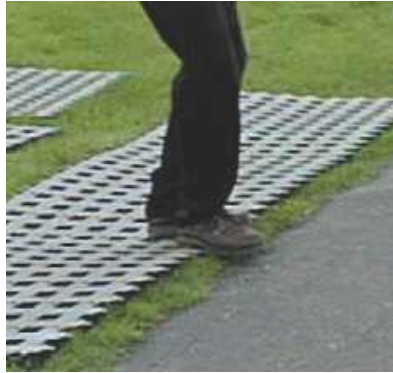
Perfo sections clipped together using foot pressure on the clips
